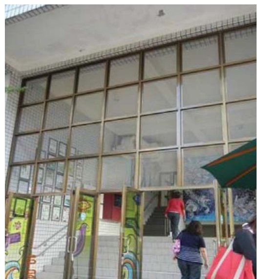
After removal of upper 2/3 glass
